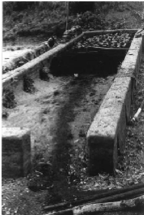
**Fig. 9.** Stall furnace for the crucible smelting of iron, partly loaded with crucibles packed in coal. Photograph by Dr. Knapp, 1936, in Hunan 湖南 province, China.<sup>17</sup>
